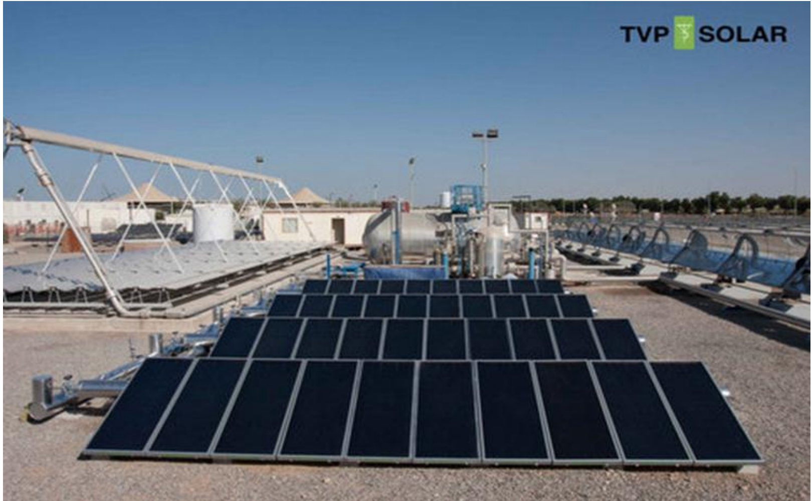
High vacuum flat-plate collector by TVP SOLAR in Masdar City (Abu-Dhabi, UAE)
